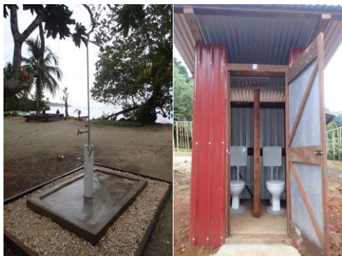
New Water Systems and toilets
