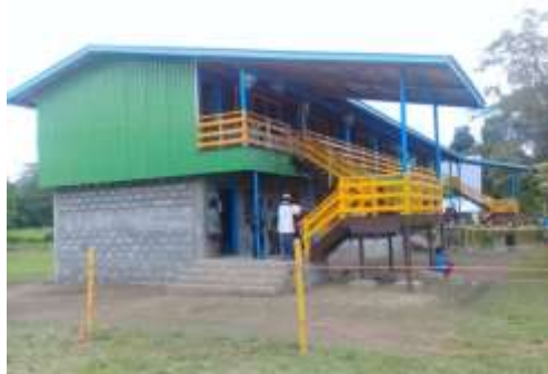
New classroom building
